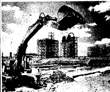
SASOL II under construction.
