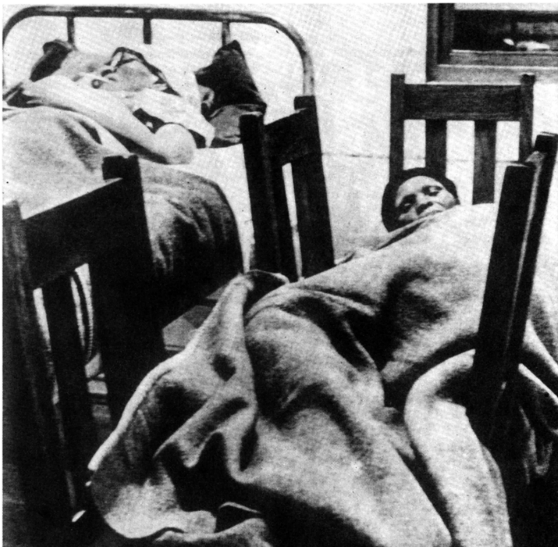
Hospital ward, South Africa
