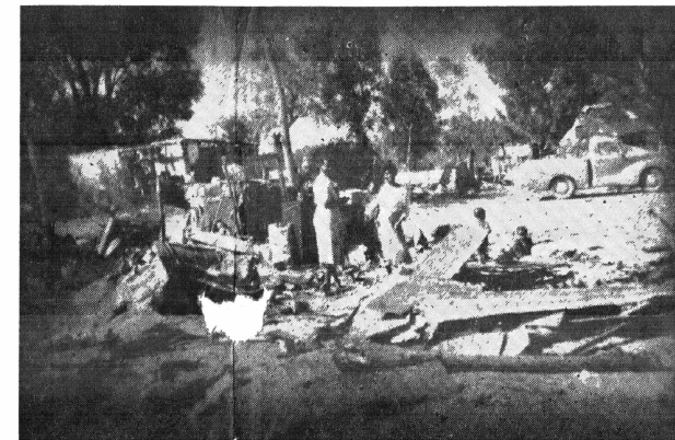
Fire damage? The aftermath of a tornado? No, this is the work of Council officials at Elsie River, destroying the homes of the people in order to force them to go to Nyanga location. Many of those whose homes were bulldozed last week told New Age they had been given no notice at all. A woman about to have a baby, and another woman with a eleven day old baby were among those who were left without any shelter for the night.
