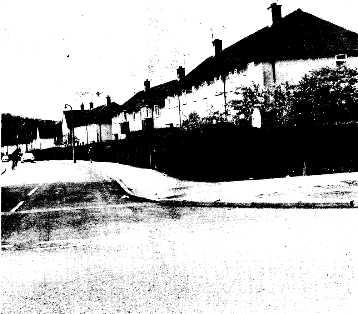
Housing on the Clifton estate in Nottingham where tenants are plagued with the problem of damp.
