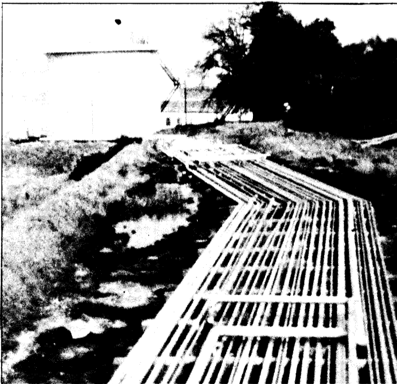
A section of the Fawley oil refinery.
