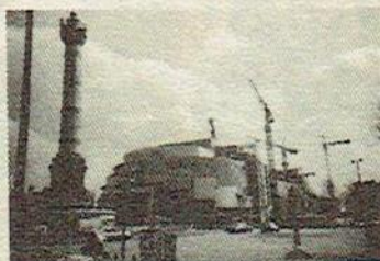
Opera Bastille under construction
