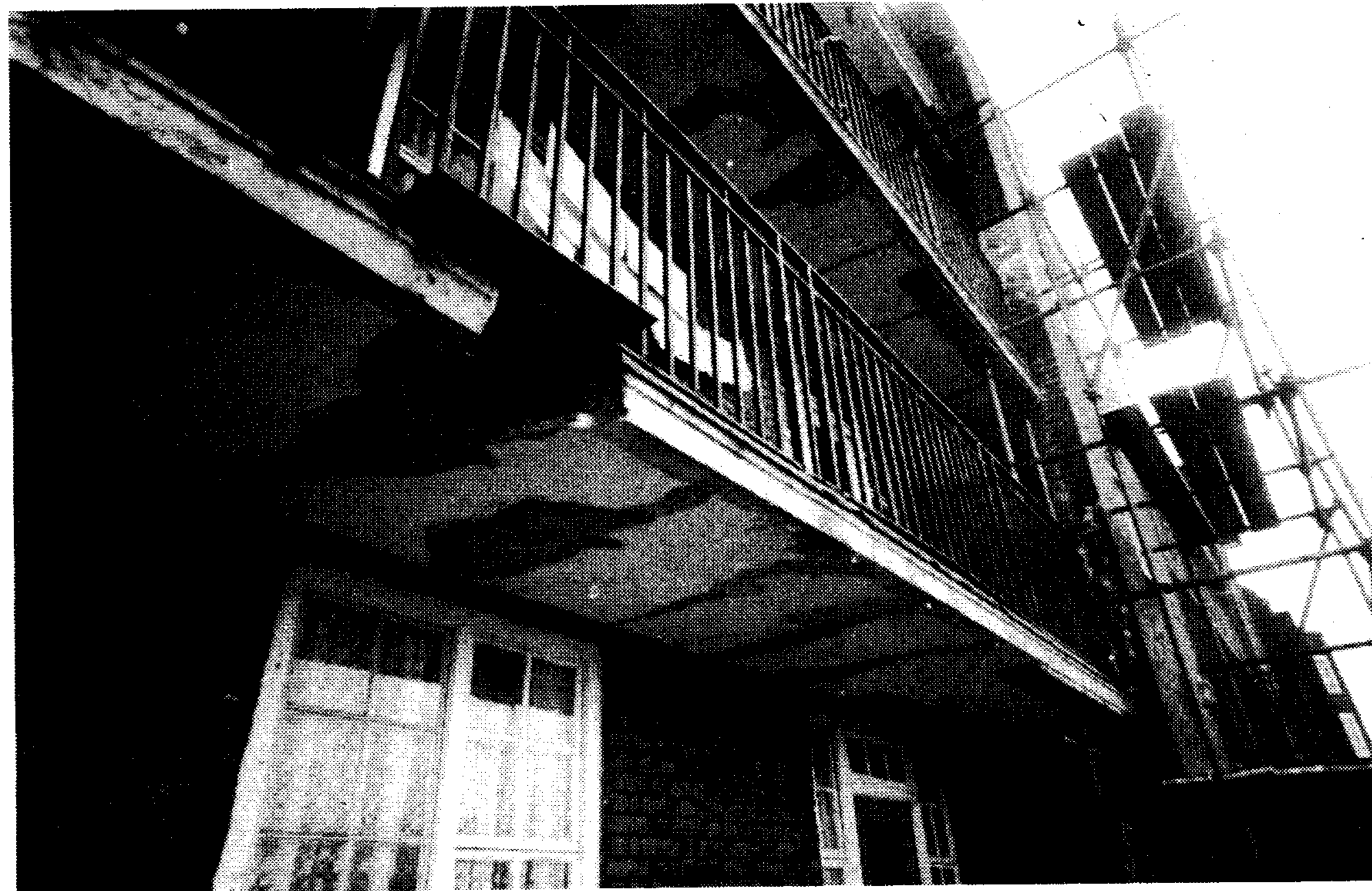
The council flats on the Isle of Dogs have been neglected for years — and now vibration from the pile drivers threatens to bring the balconies down
