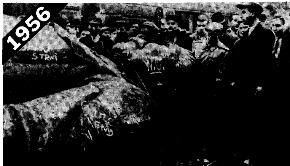
Hungarian workers demolish Stalin statue
