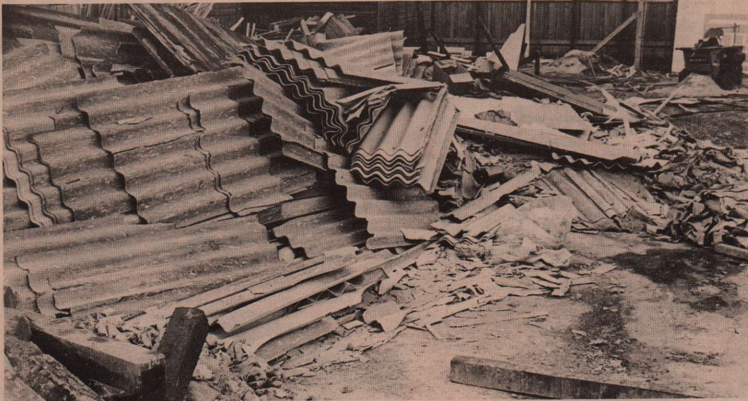
Death in the corner of the yard. Asbestos waste in a Scottish factory
