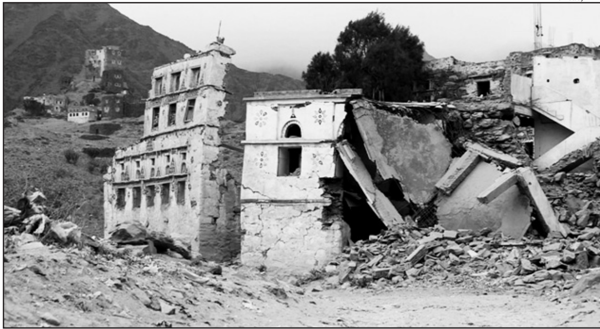
(Left) Destruction near Dammaj, northern Yemen.
