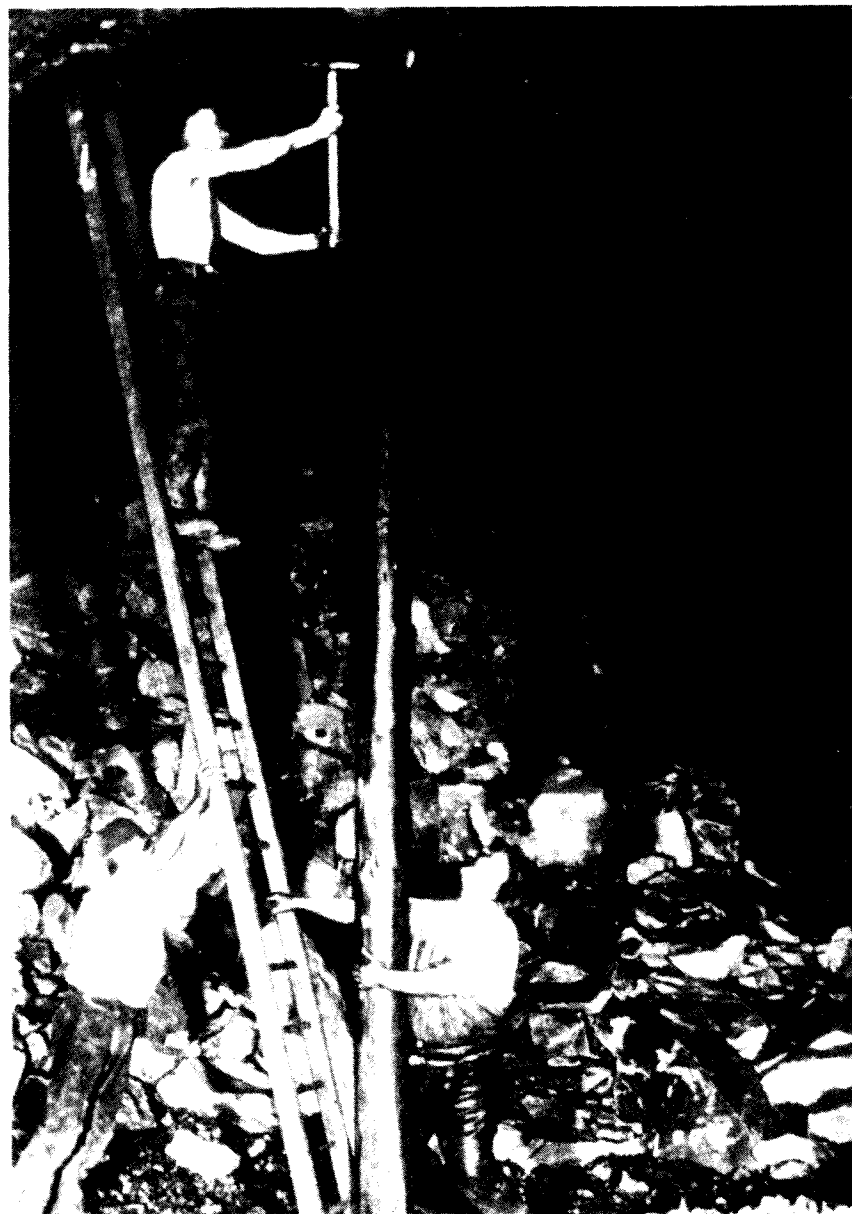
Fixing timber props at the turn of the century.
