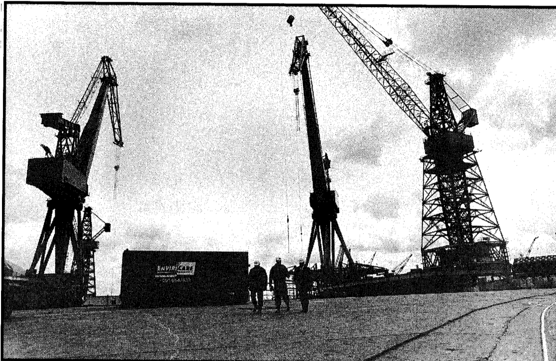
Swan Hunter must be renationalised under the workers' control
