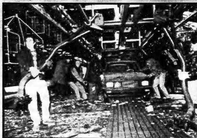
Striking Mexican students sent aid to Yugoslav workers at Zastava auto factory, here repairing production line after NATO bomb attack.
