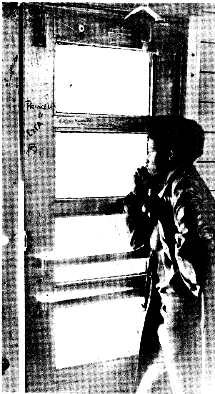
The decay in public housing services have met resistance from the tenants in Newark’s Stella Wright Project. Above: tenants show faulty plumbing and leaking pipes. Below: lobby in project.
